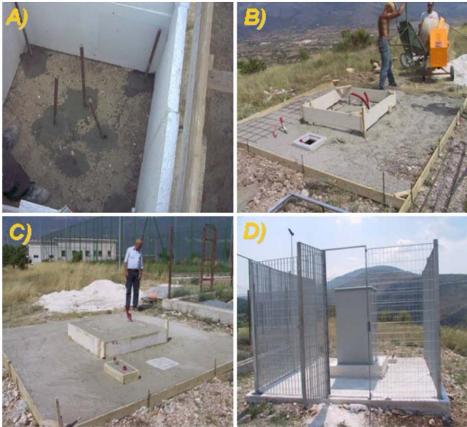
**Fig. 4** Construction planning of a standard RAN digital stations: **a** the anchorage reinforced concrete block is directly anchored to the foundation soil by means of oblique steel bars. The maximum depth of the excavation is 150cm; **b** an rc slab and cover complete the block anchorage; **c** polystyrene panels and a light floor slab guarantee the block isolation; **d** a standard fibreglass box and an external steel fence install for the station security
